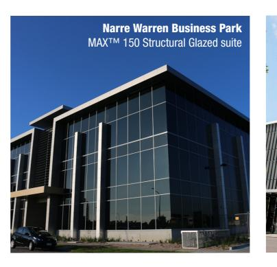
Less external metal translates to improved U-values, allowing SG systems to deliver better thermal performance over time.
